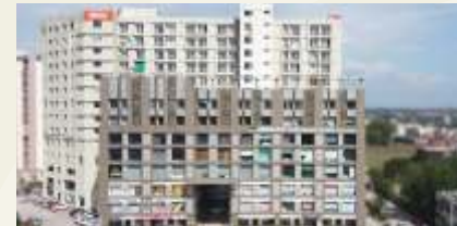
COMMERCIAL PROJECT, ZIRAKPUR
